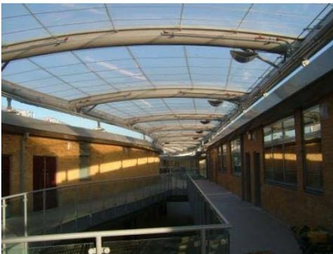
In its single ply form, ETFE foil has been used across the world. It's light weight nature, and very similar appearance to glass, means that it is frequently chosen for new buildings and old alike. An ETFE roof can be formed either by stretching the ETFE into panels as can be seen at Camellia House in Nottingham, or alternatively the membrane is supported by a cable net. Failsworth and Radclyffe schools both adopt this method in order to achieve large spans without intermediate steelwork.
