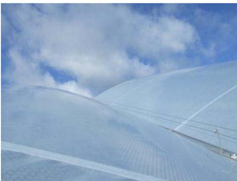
As an alternative, ETFE foil can be used to form ETFE cushions. Using inflation units the ETFE cushions provide a lightweight and insulated roof installation and can be manufactured to any shape or size, only limited by local wind or snow loadings.
