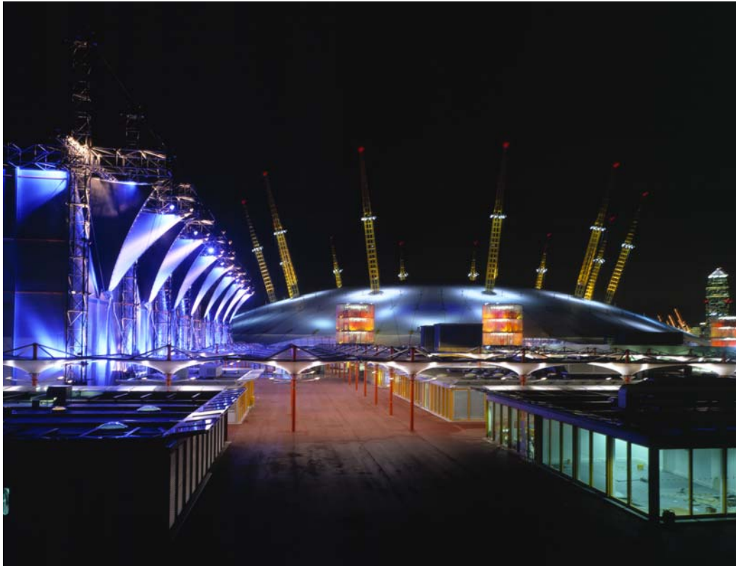
Photograph 1. The Millennium Dome, London; Skyscape is the building along the left hand side of the photograph.
