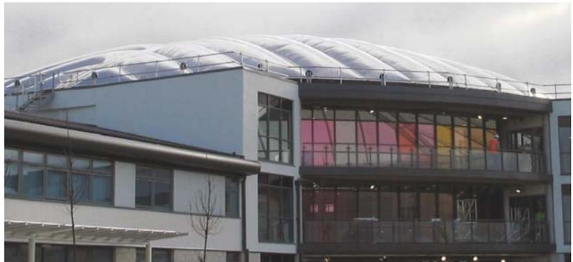
While no ETFE structures have been in place for long enough to gain a true understanding of the life cycle of the foil, the material has been extensively researched and tested in a laboratory environment and out in the field. These tests have concluded that no degradation or loss of strength has occurred and there is no sign that the material will become brittle or discolour over time. As a result, it is anticipated that the material has a life expectancy in excess of 50 years.
