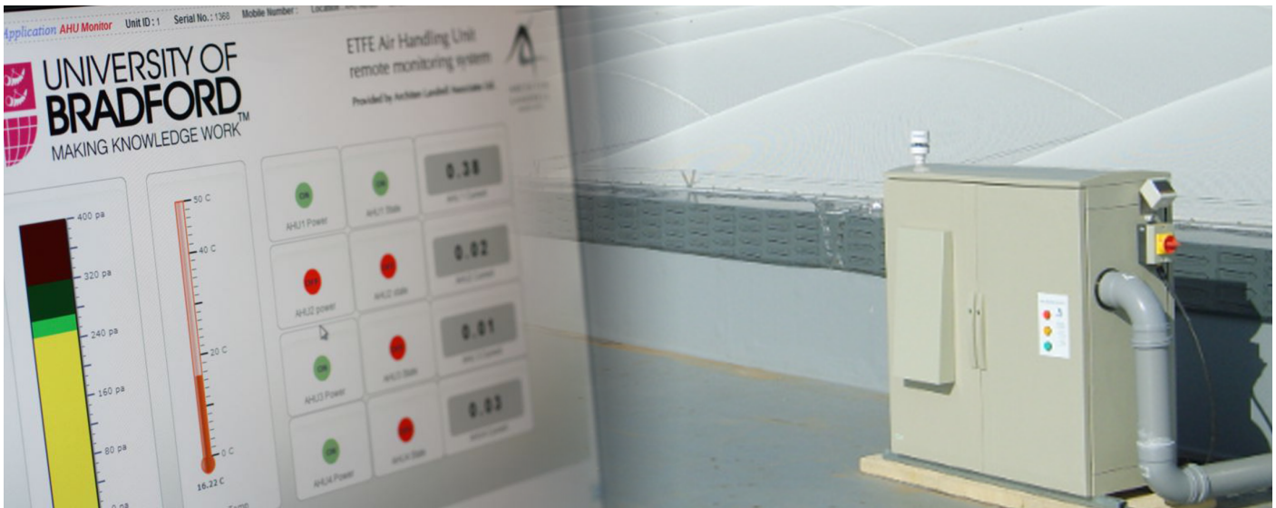
Architen Landrell ETFE Air Handling Unit with Remote Monitoring
