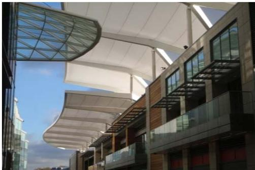
aesthetics and its high crease resistance makes it effective for demountable and retractable canopies. A good example of a Tenara structure is the Eat Street project at the Westfield Shopping Centre in London.
